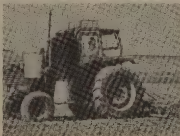
Olkkala, Finland, 1980. Wood-powered diesel tractor.
